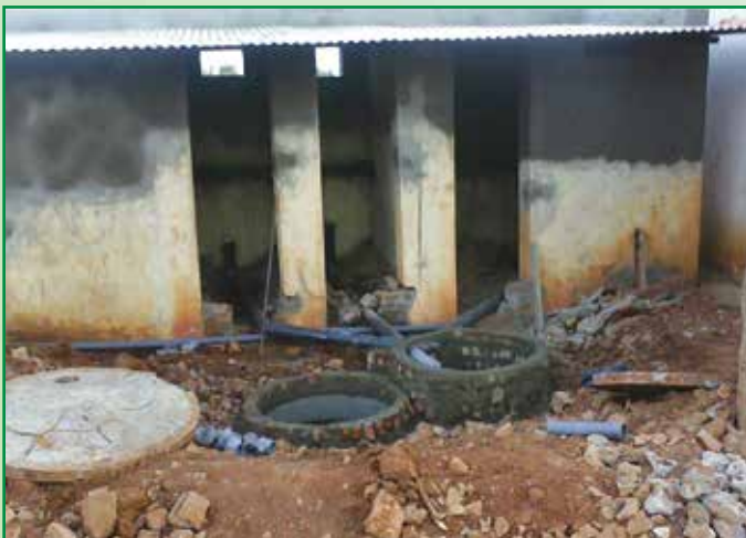
Renovation of old toilets and constructions of Sandpit
