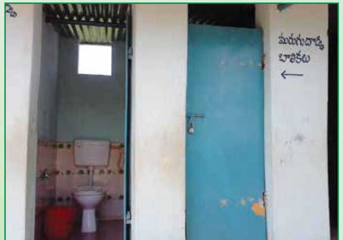
Newly done Toilets
